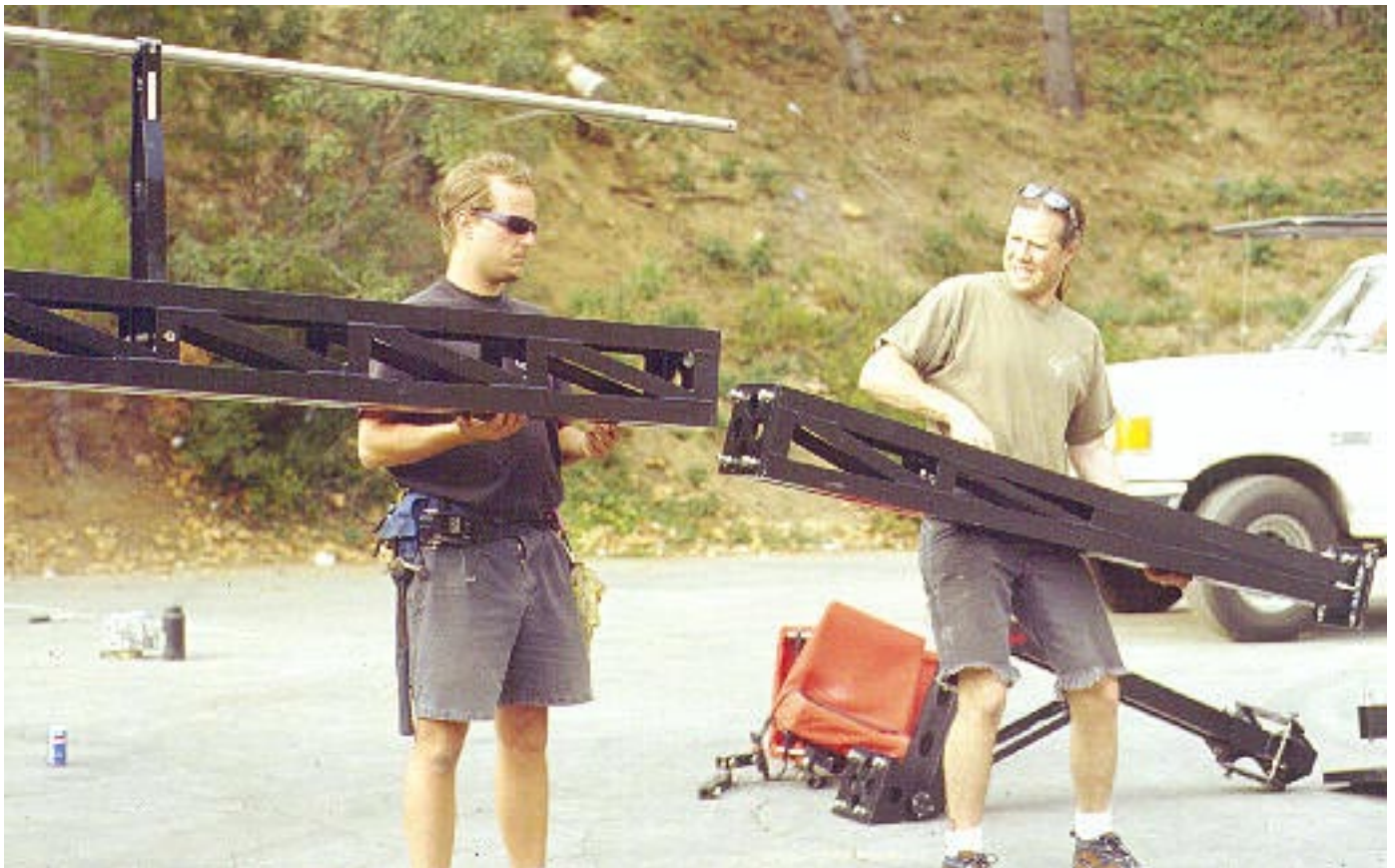
Mode 5 - Remote only - Step 18: Attach Boom #4 to the front of the Remote Boom and secure it with the 2 retaining bolts found inside the Remote Boom.
