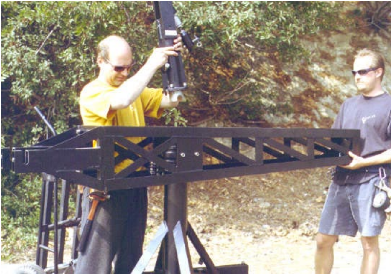
Mode 1 - Remote - Step 13: Attach Pylon assembly to mini post with 4 bolts in pylon. Horizontal shaft is then trapped into place. (Be sure that threaded end of the pylon rod section is facing towards the front- so you can level operating platform later!)
