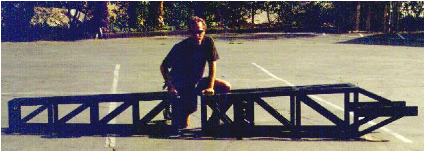
Mode 2 - Remote - Step 1: Boom #1 and Boom #2 should be assembled on the ground.
