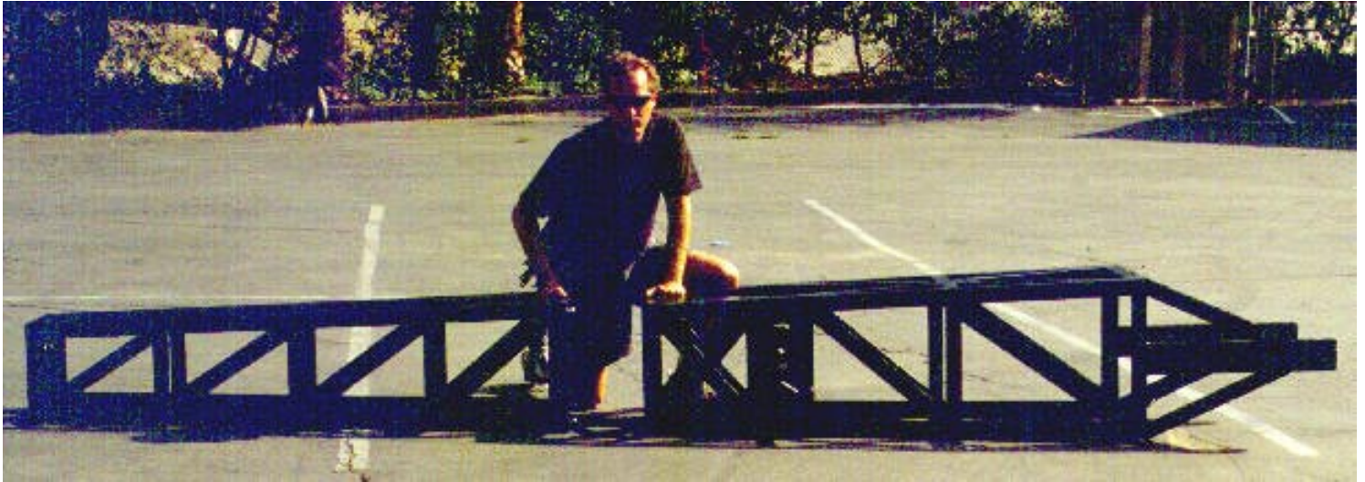
Mode 3 - Remote - Step 1: Boom #1 and Boom #2 should be assembled on the ground.
