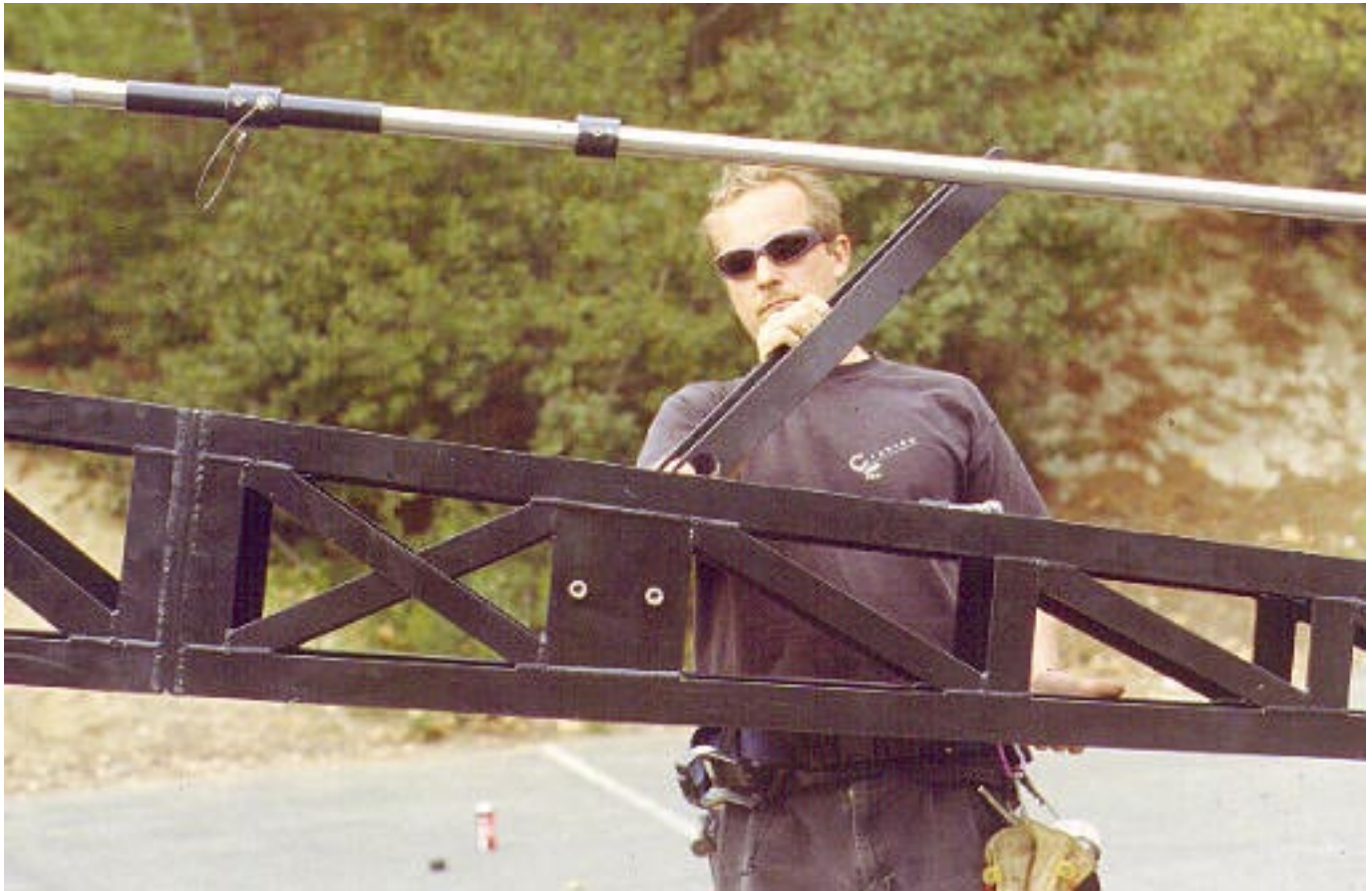
Mode 3 - Operation Platform - Step 13: Place rod support bracket over the horizontal shaft on Boom #3.
