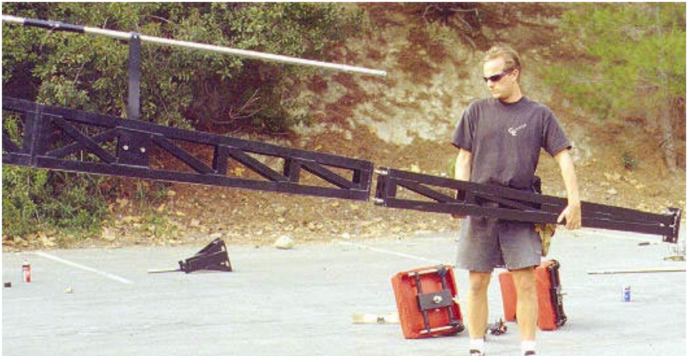
Mode 4 - Remote - Step 15: Attach Boom #4 to the front of Boom #3 and secure the 2 retaining bolts found on the inside of Boom #3.
